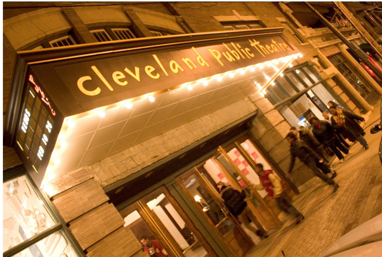
Cleveland Public Theater - Photo courtesy of Gordon Square Arts District
